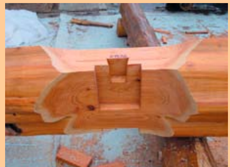
▲ Dove tail socket joinery in a roof beam
