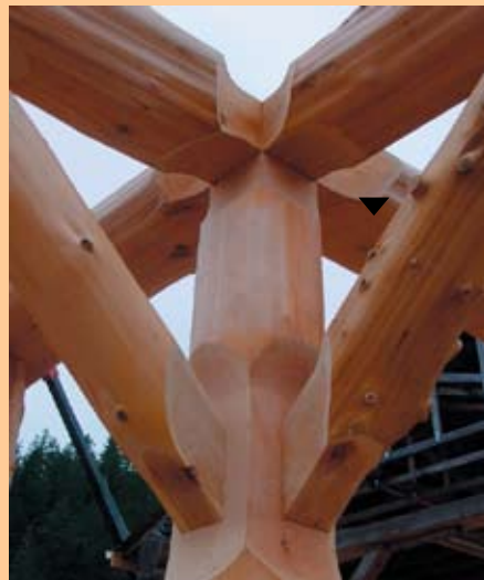
▲ Floor beams and knee braces meet a post. ▼
