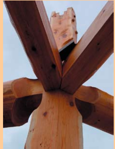
▲ Floor beams countersinking into a main post at different angles.
