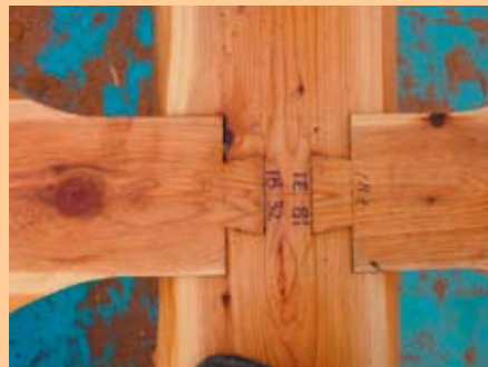
Typical floor beam connection using dove tail joinery ▼
