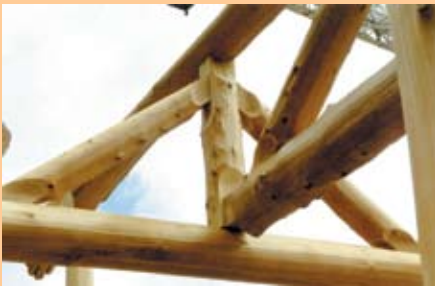
Truss systems provide wide open spaces with fewer posts. ▼
