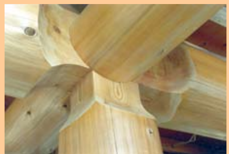
▼ Beams joining over a post.
