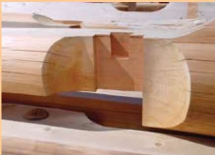
Dove tail joinery in a roof purlin ▼
