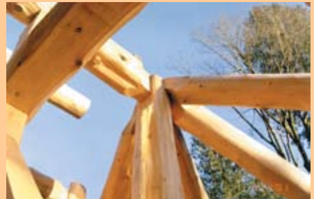
▲ Compound joinery hip rafters and ridge beam meet over a center post.
