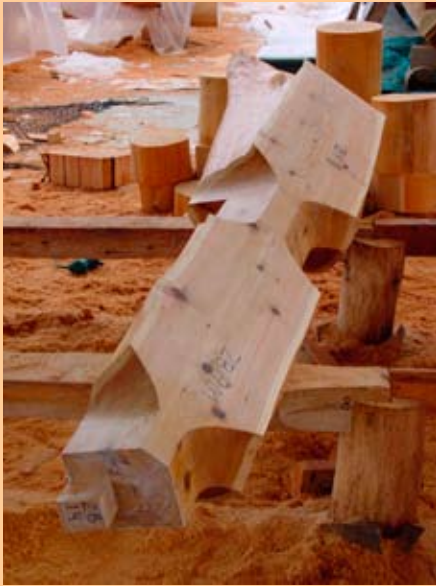
Purlin with dove tail end joinery and framing flats ◀
