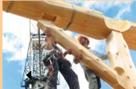
▲ Setup moment. A knee brace is being installed. No hardware is required as we use countersinks.
