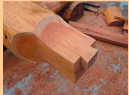
Dove tail plug end in a tie beam ▼
