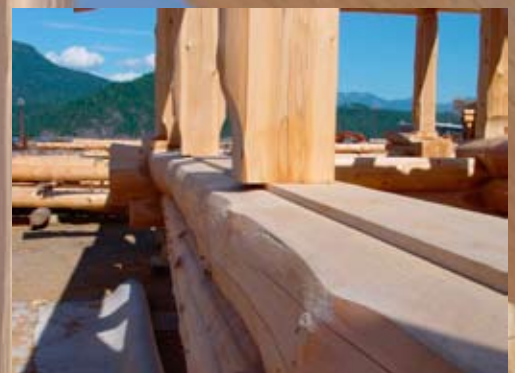
WCLH’s water shedding, stepped drip sill detail. ▶
