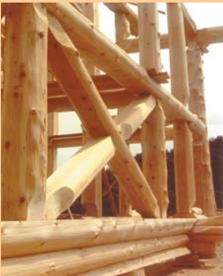
▲ X brace providing stability in an outside wall element.
