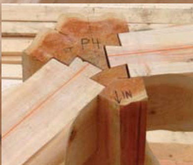
◀ A dove tail post to beam connection.
